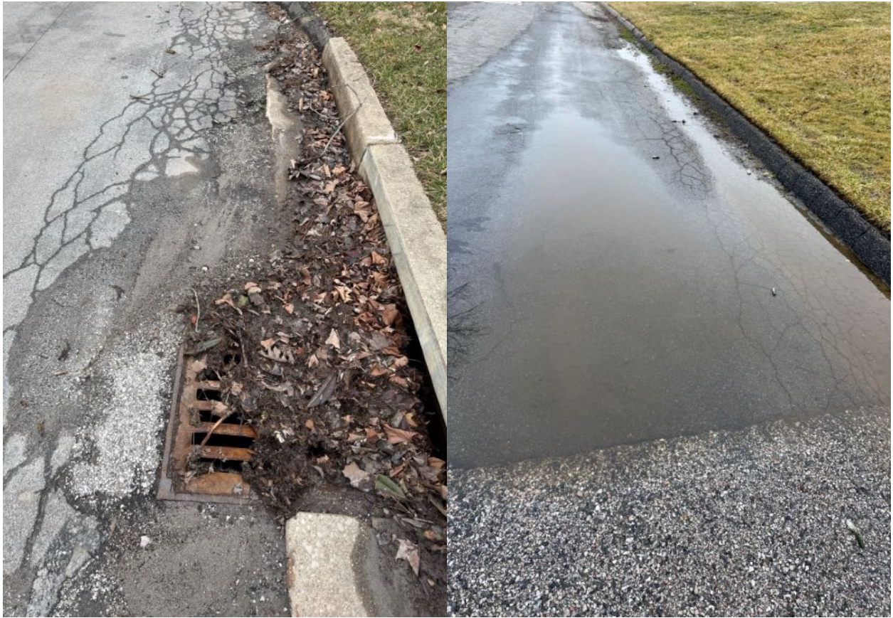
Photo showing Success of the Full-Width Repaving and Replacing Curbs in the Wyngate Neighborhood.
