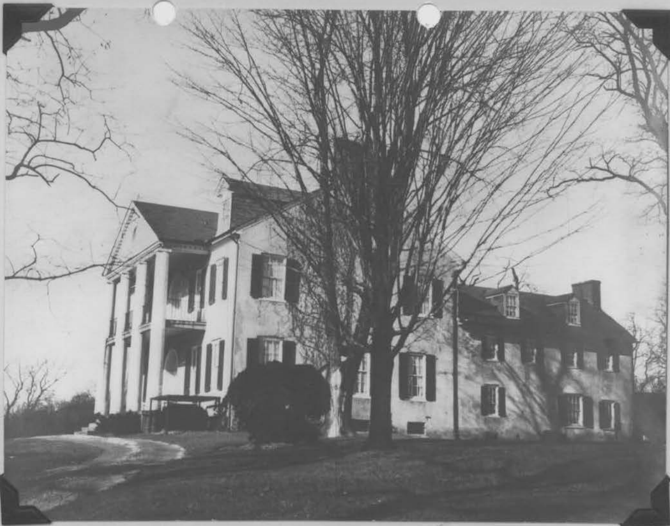
POT SPRING PRIOR TO 1936, AS IT APPEARED DURING CIVIL WAR, & PERHAPS ORIGINALLY. FRONT PORCH MAY BE ORIGINAL.
