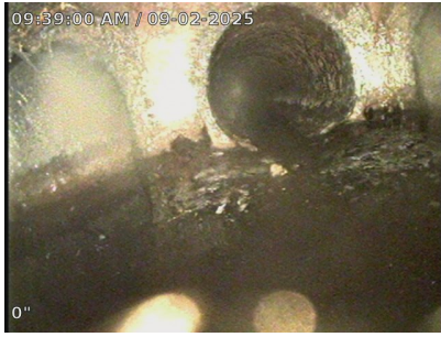
Start of video. Entry point septic tank back line toward distribution box. Video begins at the distribution box and is pushed into drainfield B. Showing distribution box.
