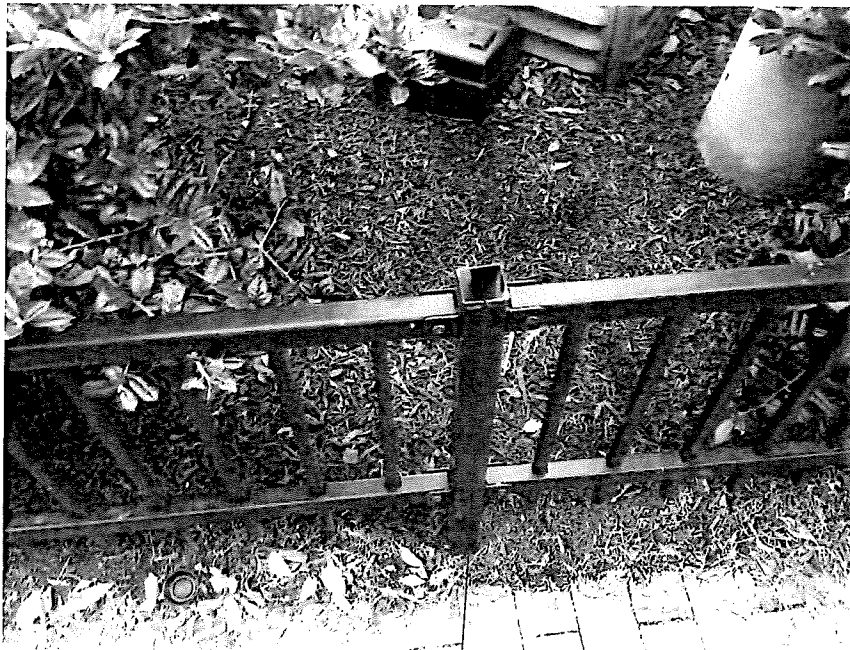
Photograph 34 – Missing fencing post cap
