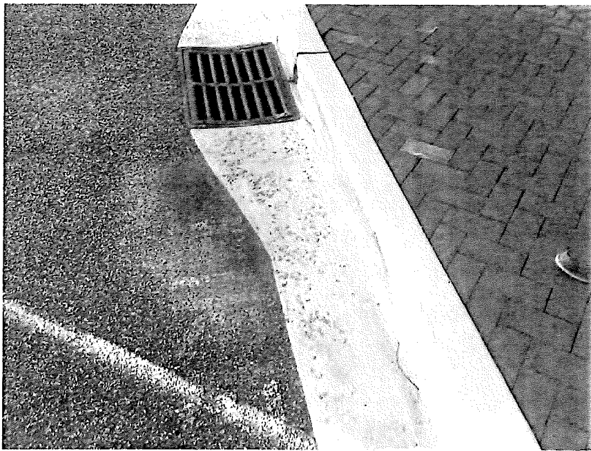
Photograph 26 – Scaled section of concrete curb and gutter assembly
