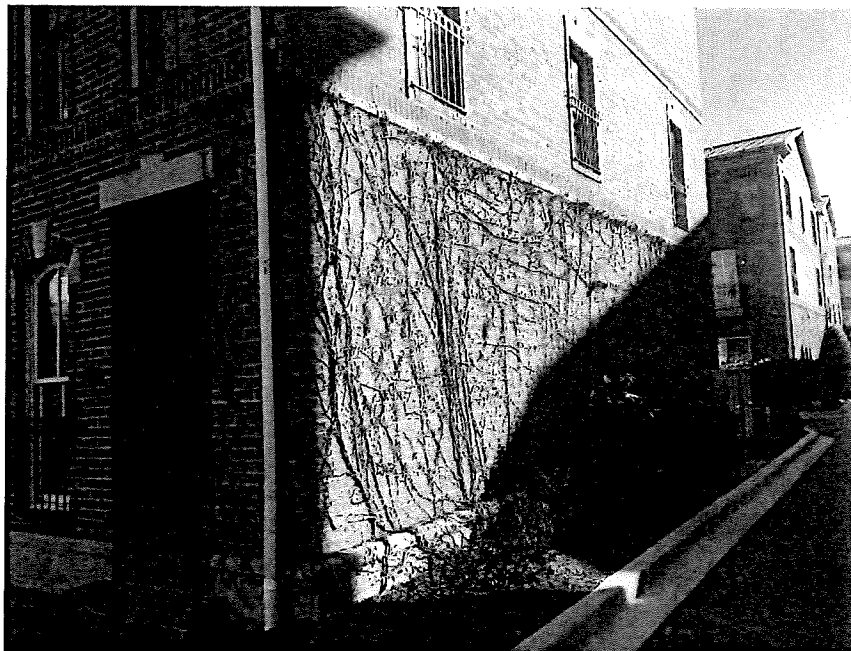
Photograph 6 – Ivy growth on brick masonry
